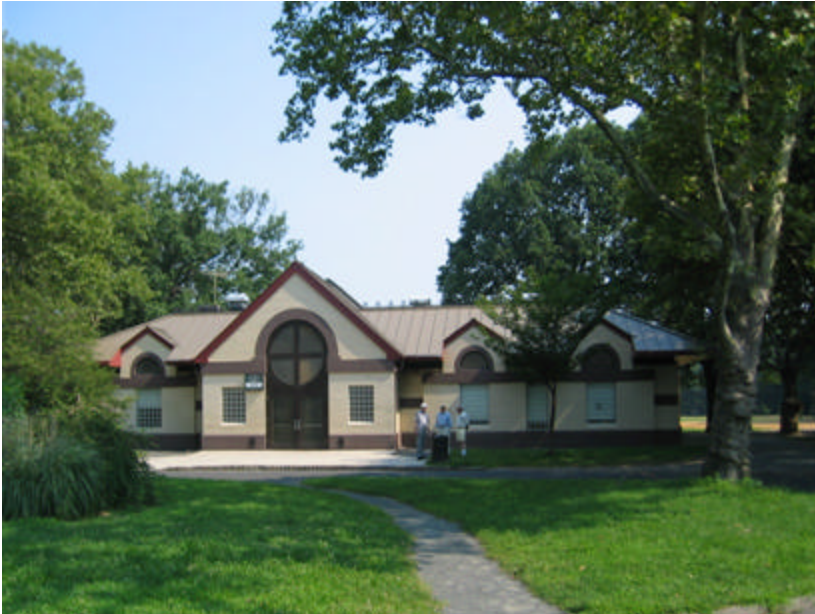
Photo 305 Overall view of the front façade.
