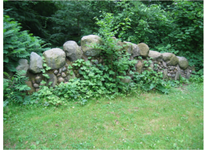
Photo 186 The south cheek wall of the bridge; note that plants are growing over most of the fieldstones.
