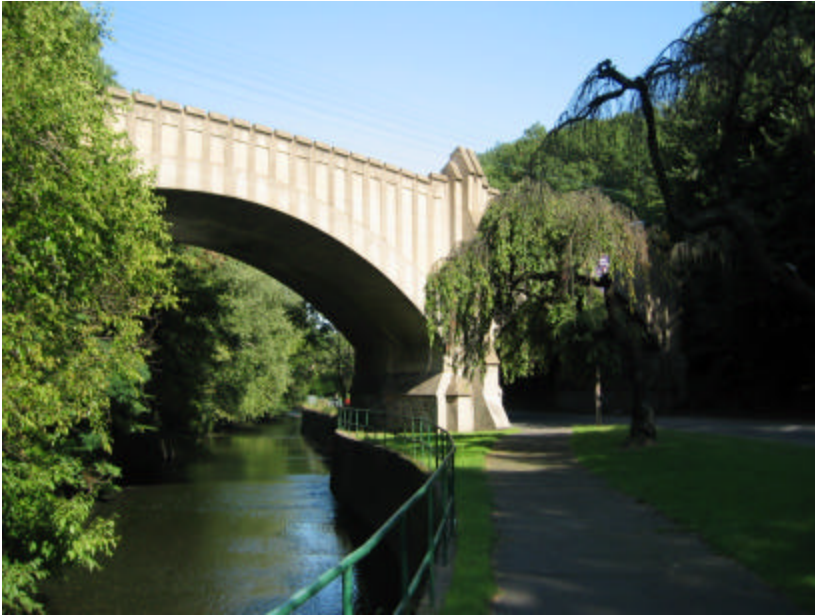
Photo 315 View east towards the bridge; note that this view of the park represents areas that are well maintained.
