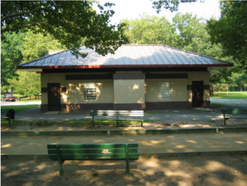
Photo 307 View of the hip roof from the bocce courts.
