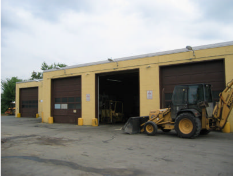
Photo 284 View of Small Garage.
