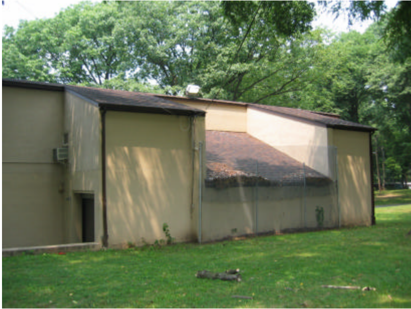
Photo 287 The sloped roof on the east side of the building; note that a fence has been placed there to prevent injury/vandalism.
