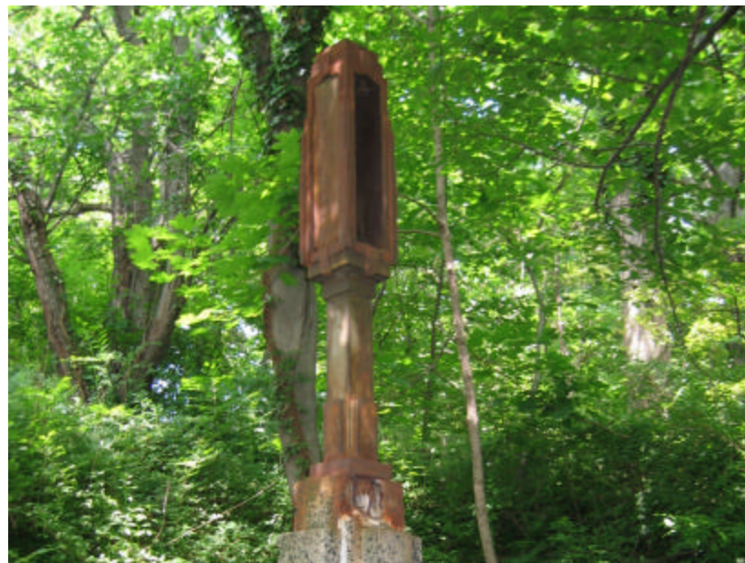
Photo 297 An original metal lantern atop a concrete base; note that the surface is severely rusted.
