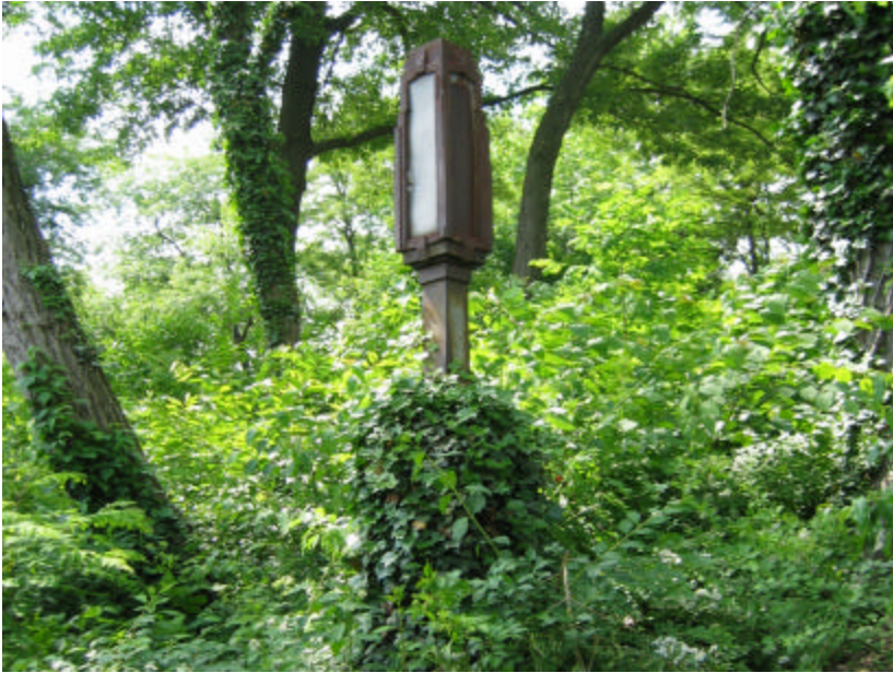
Photo 300 The base of this lantern and the entire area is covered with vegetation.
