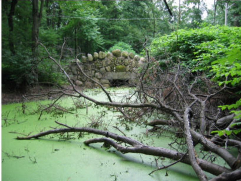
Photo 189 The north cheek wall of the bridge showing the flat granite lintel that spans the opening to the concrete underside; note the significant amount of debris and vegetation around the site and the sediment deposits under the bridge covering the original rock work.
