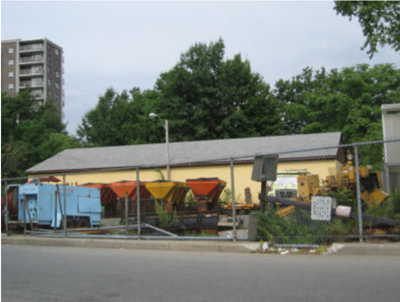
Photo 278 View of the Maintenance Facility site showing chain link fence along Park Drive and the badly damaged concrete curb; note the extensive array of material and equipment visible from the Park.
