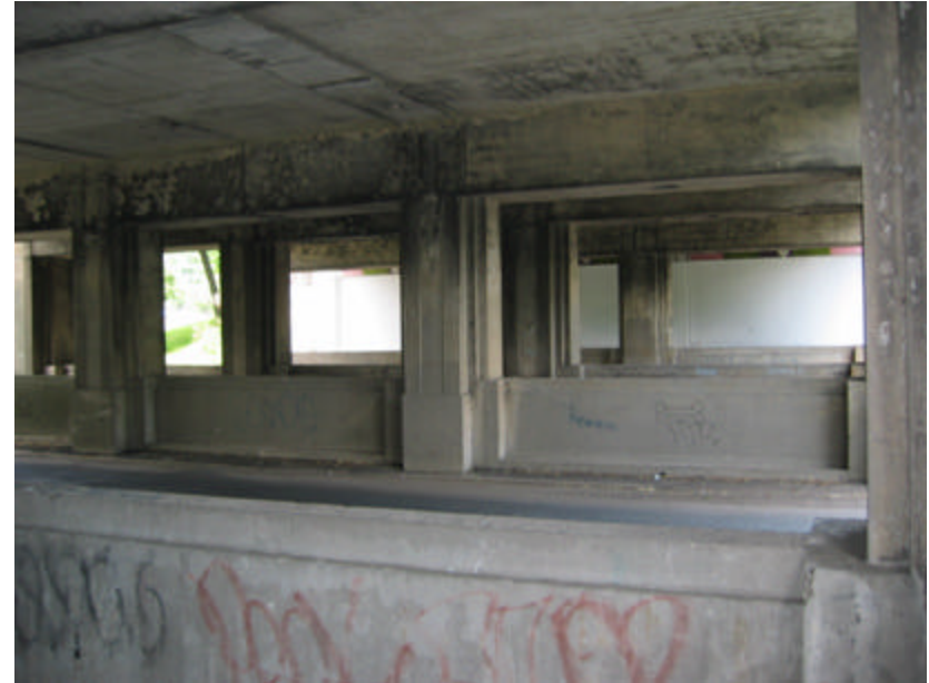
Photo 299 View east underneath the bridge; note the graffiti and soiled surfaces.
