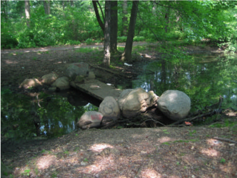
Photo 195 Weir 2 is constructed from concrete and has boulders set into concrete on each side.
