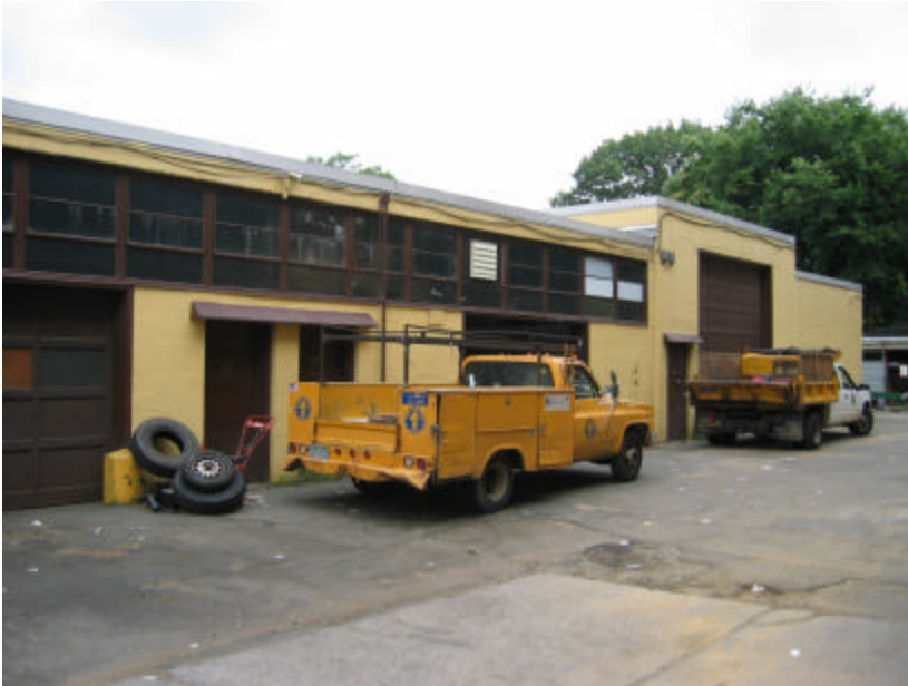
Photo 282 View of east wall of the main Maintenance Garage; note that the continuous "clerestory" window provides significant natural light.
