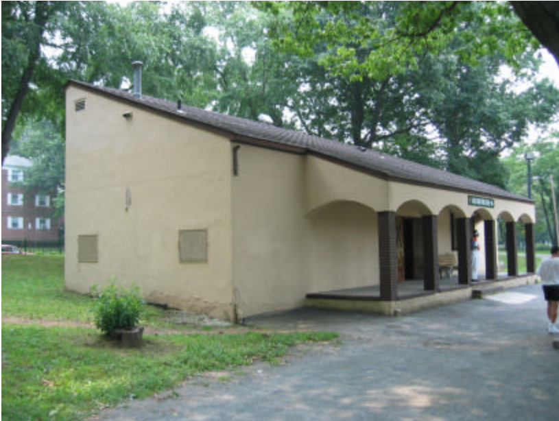
Photo 285 Overall view of the tennis center; note the arched porch.
