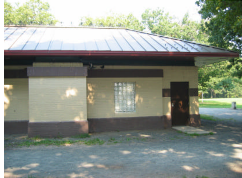
Photo 310 The dark brown concrete belt course; note the pigeons resting on top of it and the areas of staining by bird excrement.
