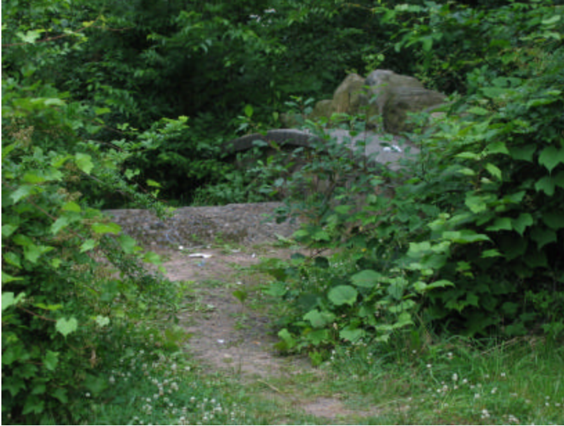
Photo 178 View east towards the Midwood Pool Bridge; note the vegetation including, trees, bushes and vines overgrowing the site.
