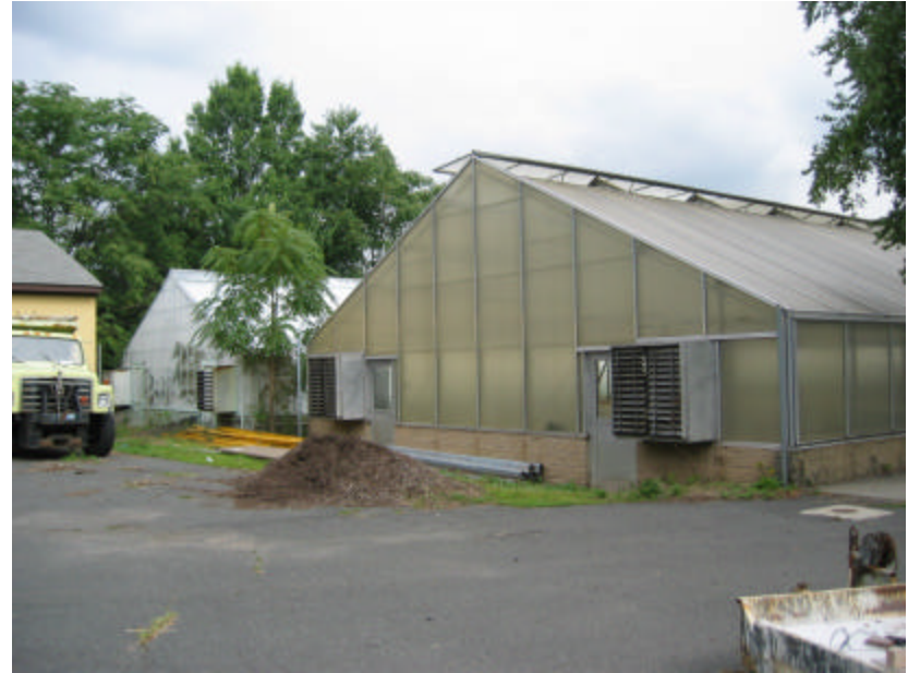
Photo 281 View of the southern gable ends of the greenhouses; note that the aluminum mullions and plastic glazing are generally low-maintenance.
