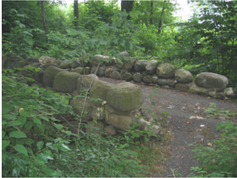
Photo 258 The Brookside Meadow Bridge; note overgrown vegetation around the site and the eroded dirt and gravel pathway.
