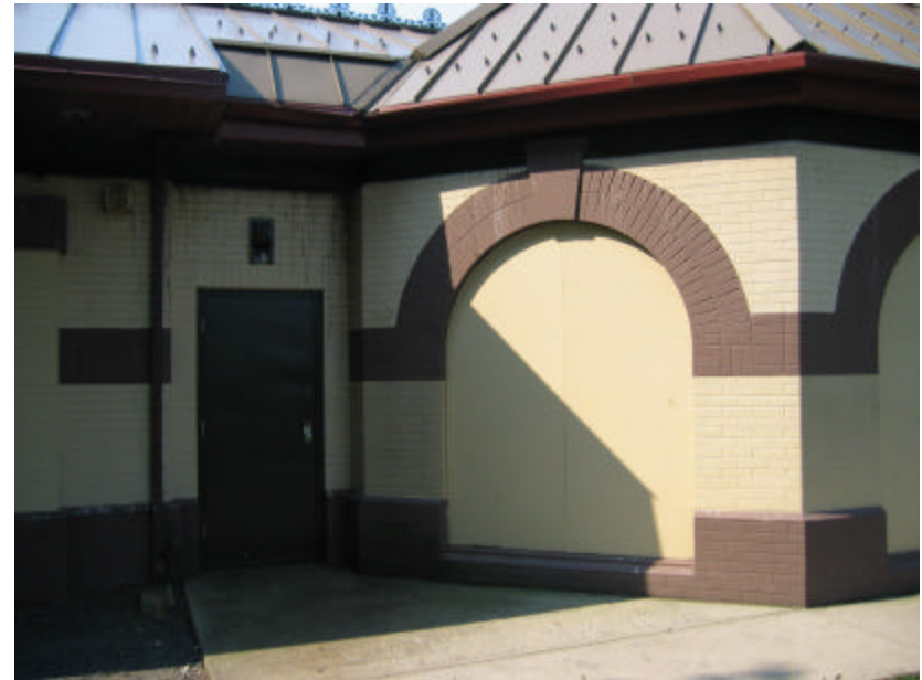
Photo 314 Large arched windows or doorways on the rear of the building; note that they are now covered with plywood.
