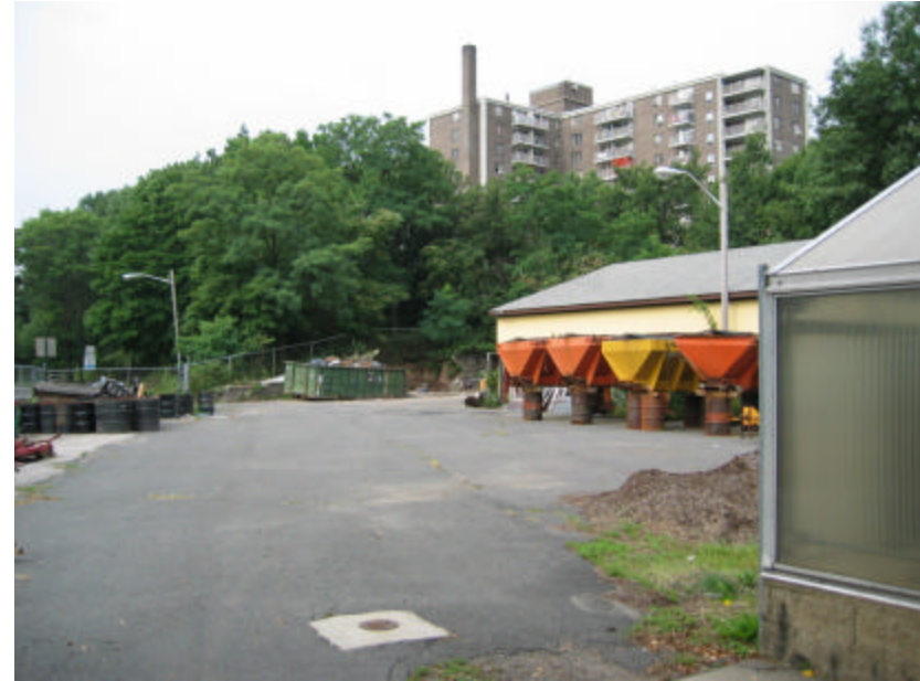
Photo 279 View of the Maintenance Facility, with the Storage Building beyond; note the southern site fence rising into the trees.
