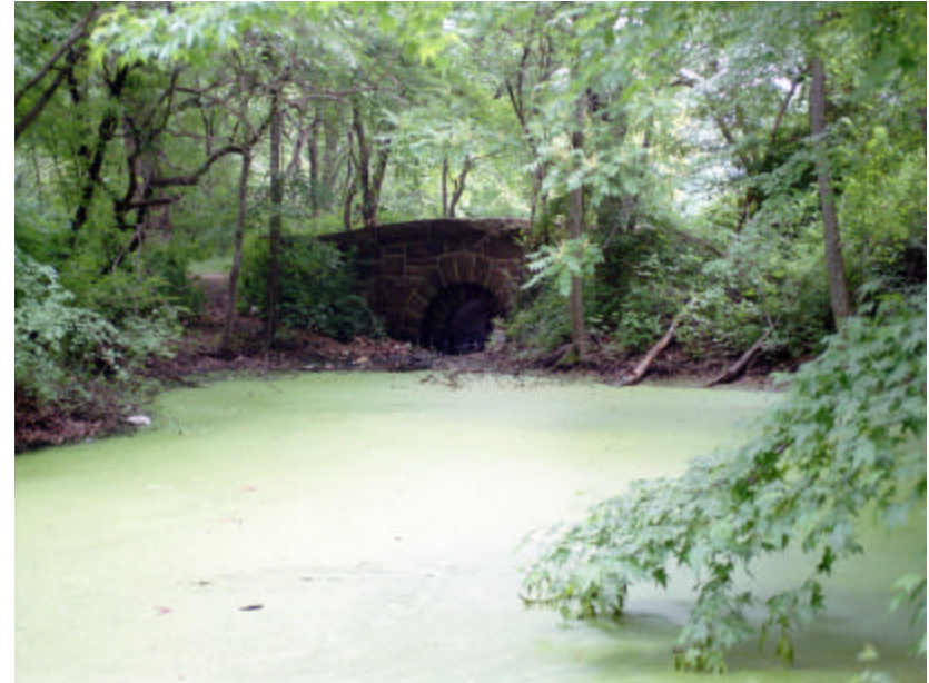
Photo 200 The brownstone bench bridge north of the Edgewood pool.
