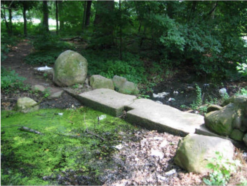
Photo 253 The fourth weir is constructed from concrete and also has a pipe that serves as a drain at its base.
