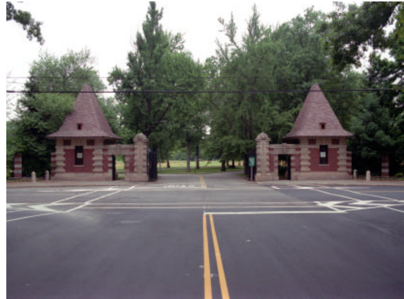
Photo 213 View of the gate from Ballantine Parkway.
