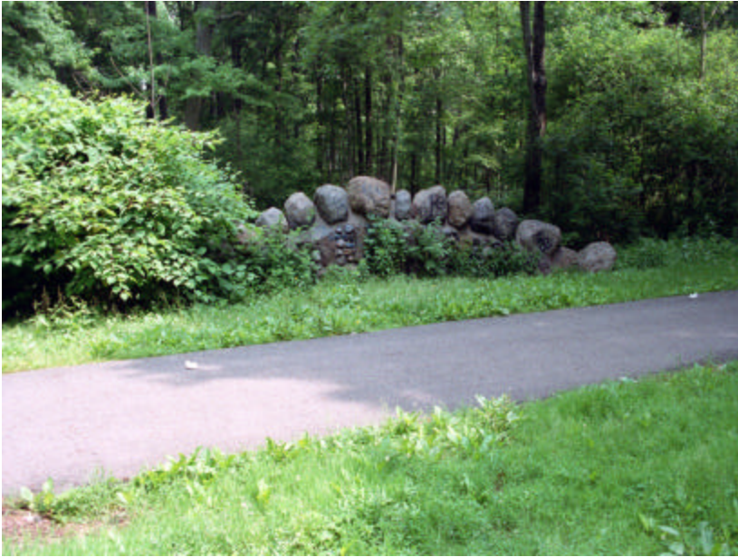
Photo 185 Asphalt path and grass-covered areas between the cheek walls; note the width of the bridge and the good condition of the pathway.
