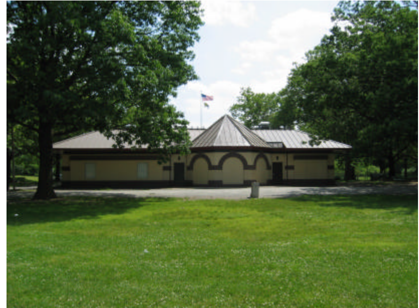
Photo 306 Overall view of the rear façade from one of the baseball fields.
